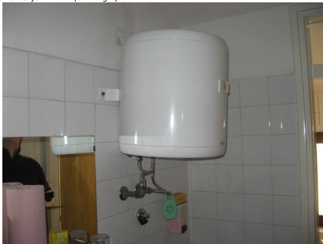
Electric heater for DHW 2 (building A)
