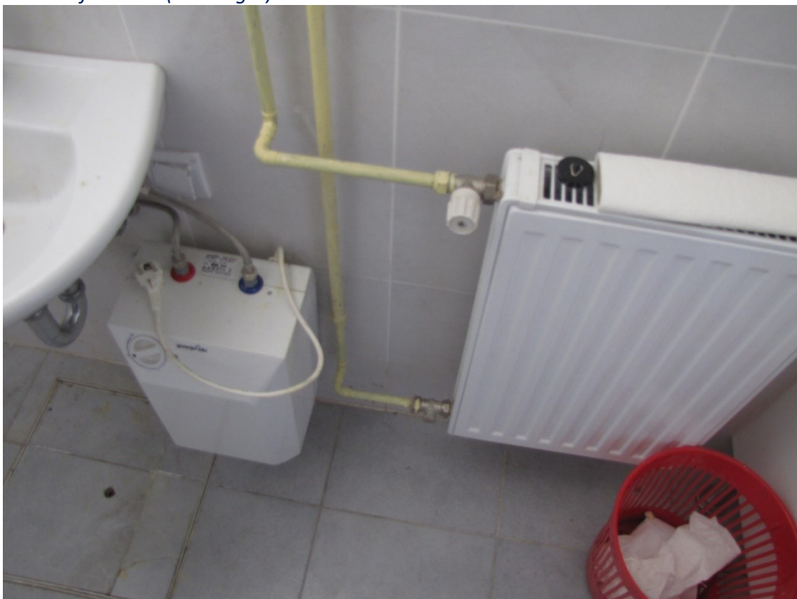
Electric heater for DHW (building A)
