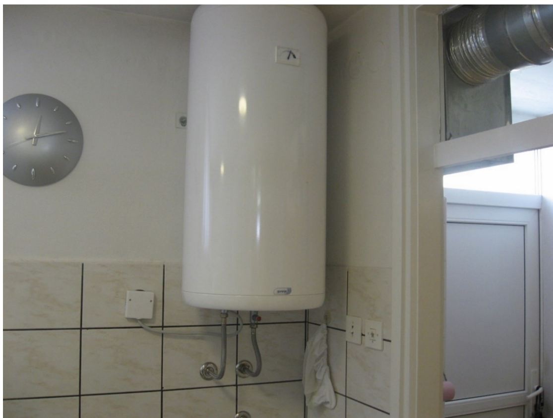
Electric heater for DHW 2 (building A)
